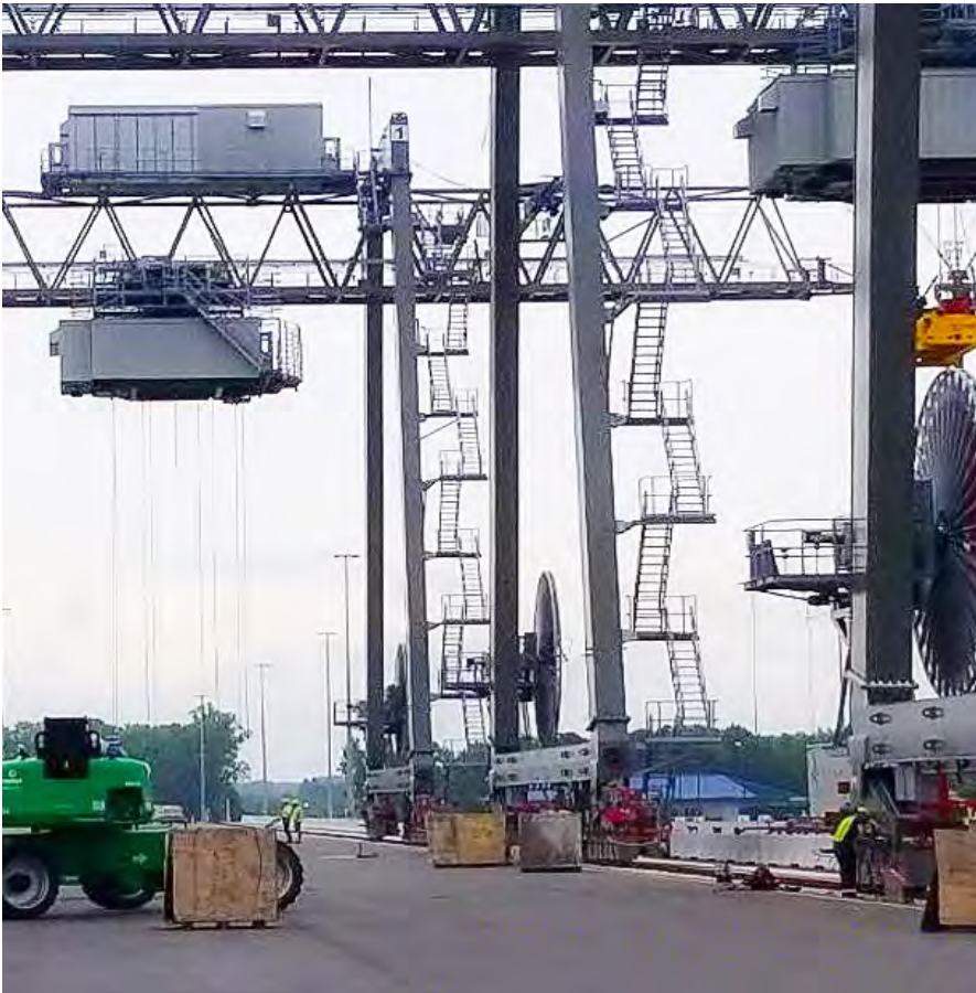
Spreader cabling for Crane 3 installed
