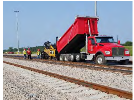
Lane paving between tracks 2 and 3
